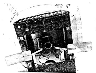
Rolleiflex SLX with reseau in cardanic suspension
