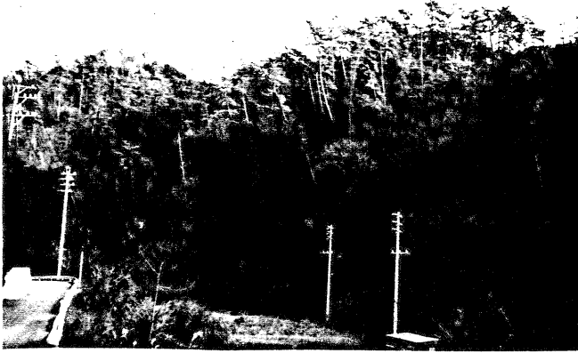
(a) Heavily damaged
