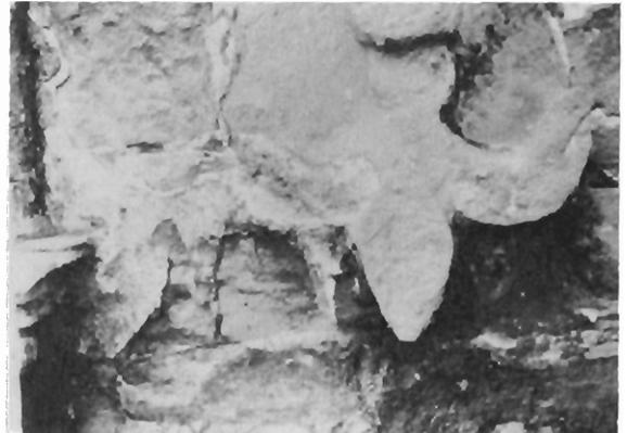
Fig.5 Details of stone damages at the upper gable of the church
