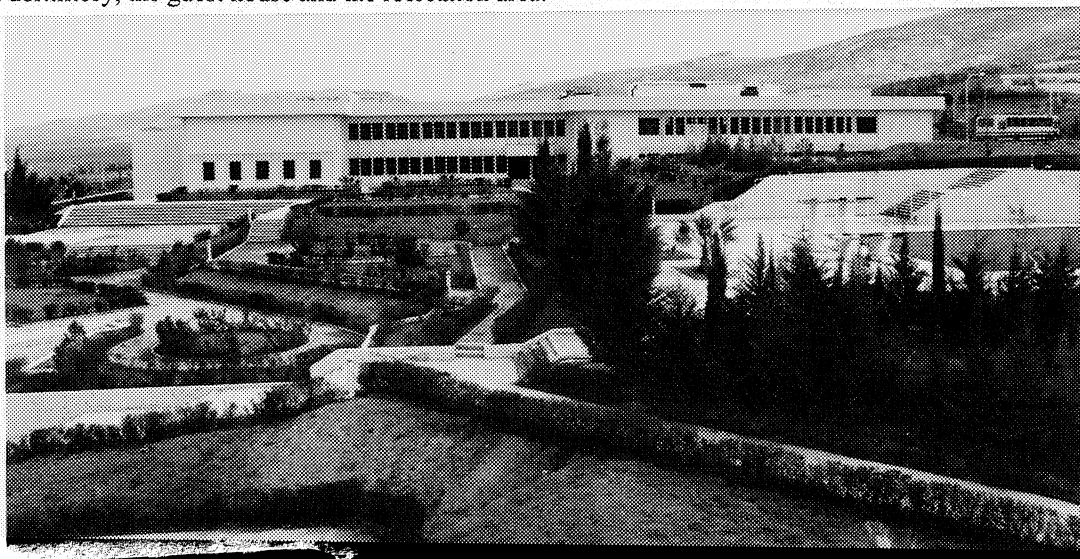
Figure1. Buildings of GORS.
