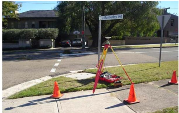
Figure 2. GCP Surveying using GPS
