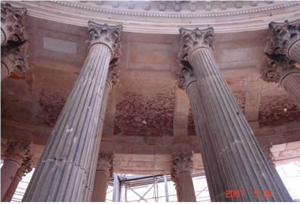
Figure 10. Actual conditions of the structure
