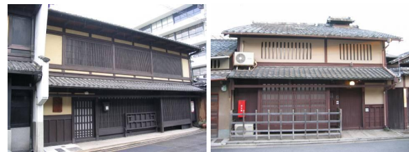
Figure 4. Typical machiyas in Kyoto (left: So-nikai or full 2 story, right: Chu-nikai or lower 2 story)
