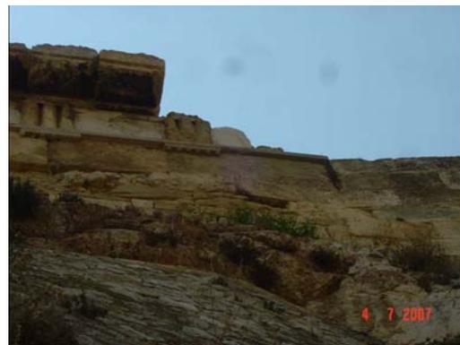
Figure 2. North part of Acropolis circuit wall. Characteristic displacements of structural blocks. By D. Egglezos
