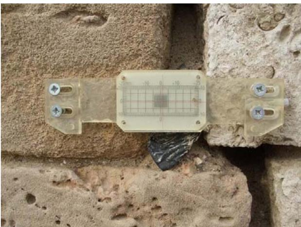
Figure 4. South part of Acropolis circuit wall. Characteristic dislocations of joints of structural blocks. By D. Egglezos
