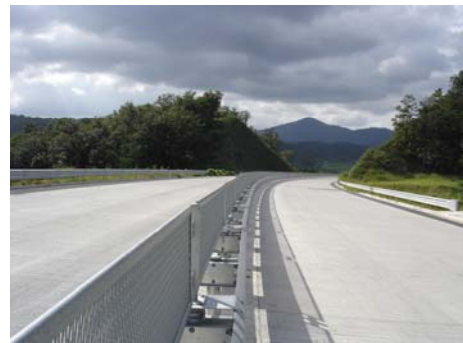
Figure 4. Photo view of test-field area
