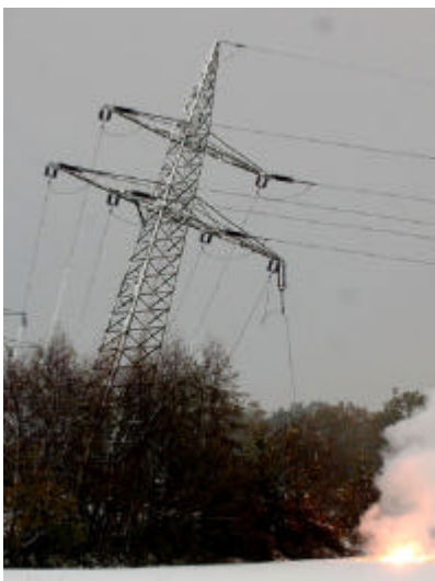
Figure 11: A pylon of a power line close to its break down in Winter 05/06 in the NW of Germany [www.wdr.de, accessed on 4.4.08]
